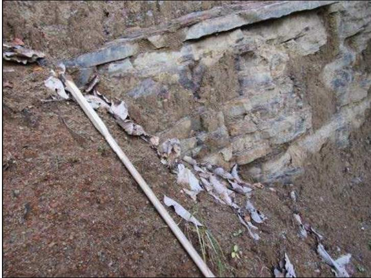
岩盤は新第三系振迫層の砂岩・泥岩互層(N25° E19° ESE、N4° E24° E、N45° E14° SE、N40° E19° SEで流れ盤)
